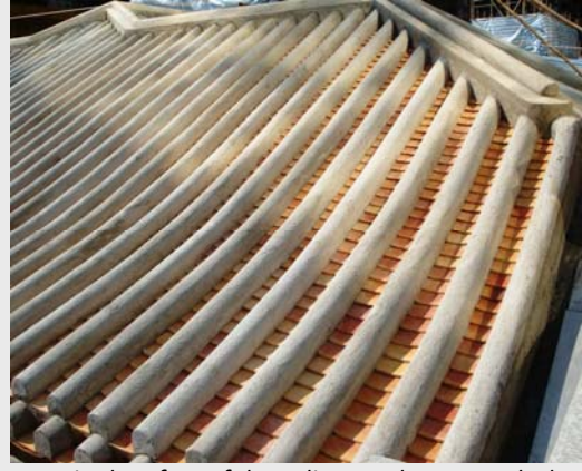
Repaired rooftop of the Police Headquarters Block
