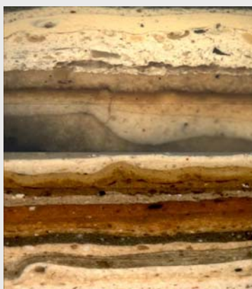
A microscopic view of multiple layers of paint with a total thickness of approximately 1.2mm on a wall surface at CPS
