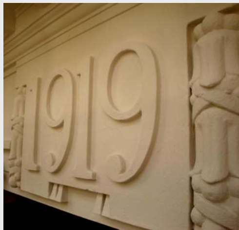
The original beige colour is restored to the exterior wall of the Police Headquarters Block
